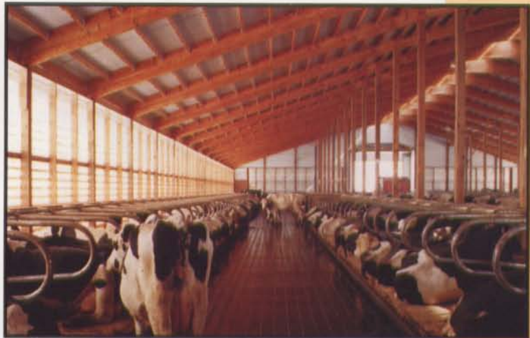
Scott and Michelle Herber's Shadey Crest Dairy, Altura, MN. Scott reported that with JanAire, they are able to use their flush system all winter - it does not freeze up!
